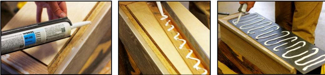
If you are using additional fastening methods, locate the fasteners in a pattern on the final 2" of the tongue. Use a pattern of placing fastener every 8" leaving 4" spaces on each end of the profile. (Refrain from fastening along the edge of the drop area.) Remember to also adhere the profile along the back corner (underside) of the profile's nosing section.
