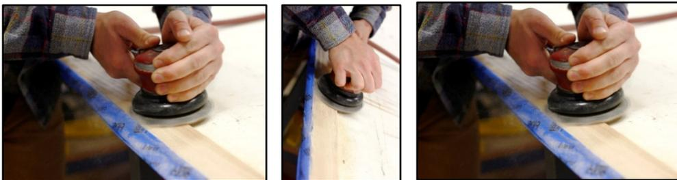
Lastly, in all cases use **painter's tape** (we highly recommend Scotch 3M #2090) for securing all profiles and flooring until final curing – usually 24 hours.
