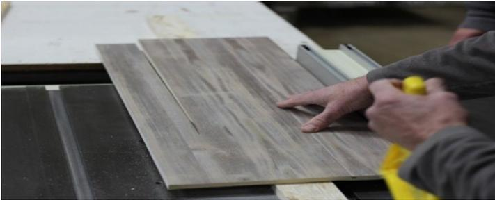
7. To assure a proper tread fit, make the width cut slightly larger than the distance from the measurement of the run by at least an 1/8". This will assure you have enough width to your tread and ensure a tight fit against the riser.
