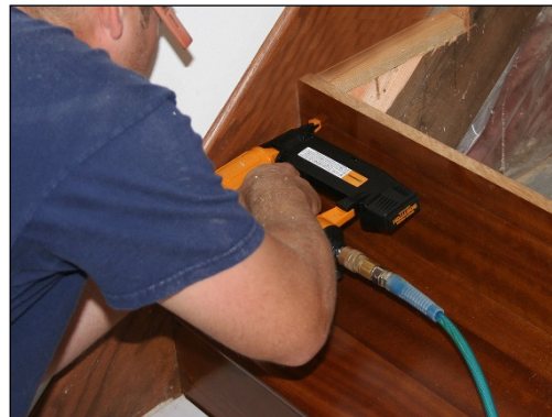
Nail the riser face into the stringer.
